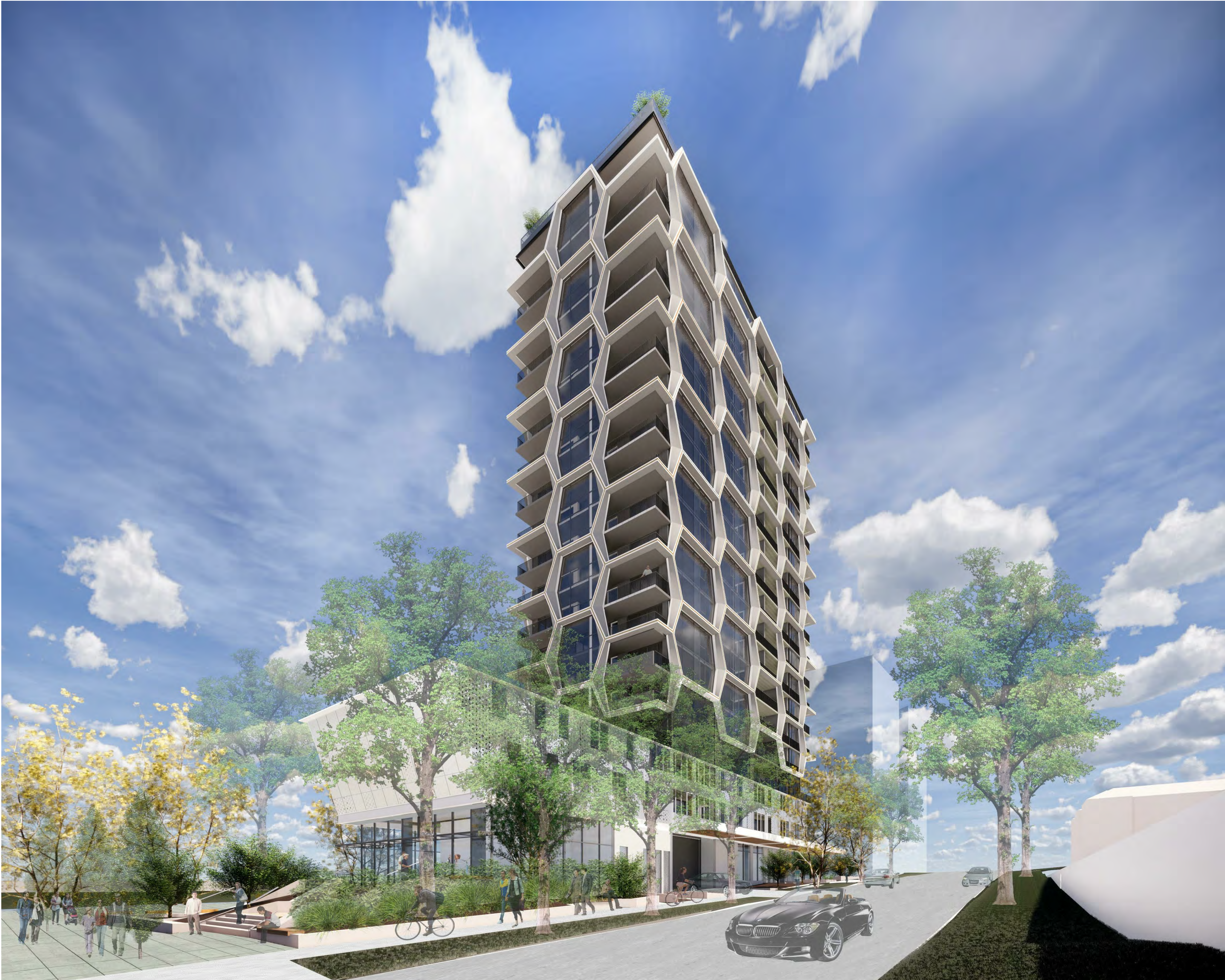
VIEW FROM COTTONWOOD CRESCENT
